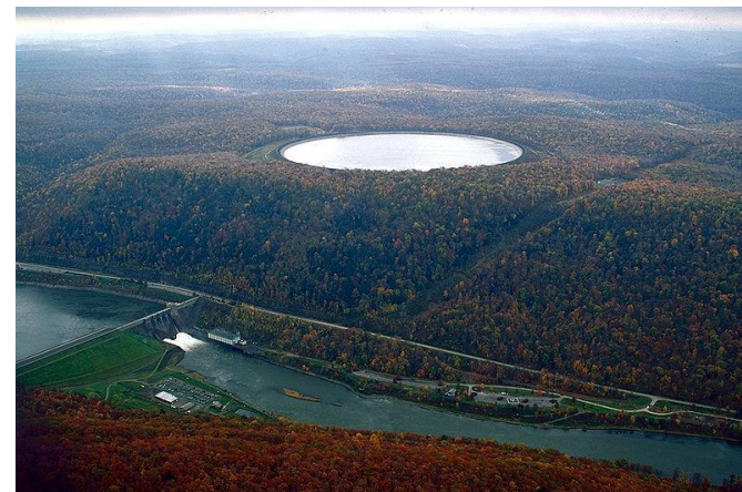
Figure: Seneca Pumped Hydro Station near Warren Pennsylvania.
